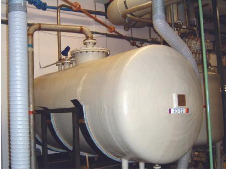
In order to protect the surrounding water supply system, industrial wastewater must be neutralized before discharge. A neutralization reaction occurs when acid or alkaline reagents are added into a tank containing waste water. Sulfuric acid, sodium hydroxide and calcium carbonate are the most commonly used reagents.
